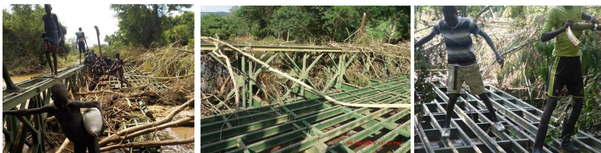
Figure 4: Damage caused by the flood on the motor bridge and volunteers cleaning the debris
